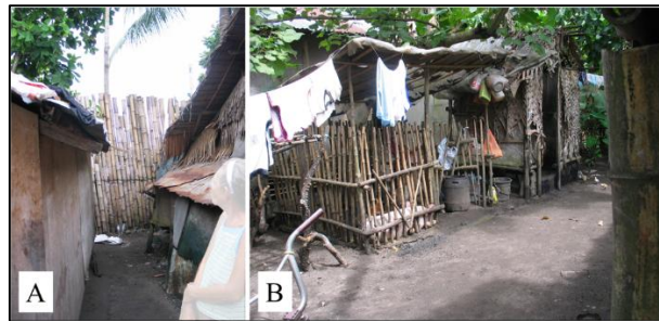
Fig 1: Bamboo housing in the Philippines. A: Bamboo windbreak. B: Bamboo livestock enclosure
